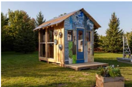
Skyhill Collective's The Textured Structure is made up of four different low-tech and accessible building techniques / photo Will Pemulis
